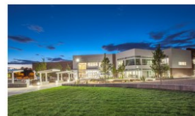
Renovation CNM Smith Brasher Hall
