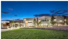
Renovation CNM Smith Brasher Hall
